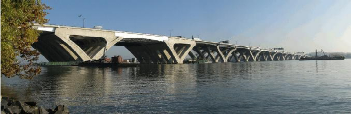
The new Wilson Bridge taking on a new form. (Photos by Ned Rhodes, photo editing by Tom Coldwell.)
