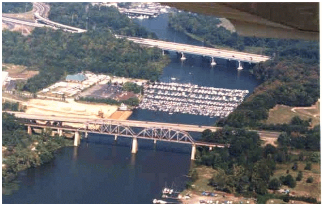
Occoquan Harbour Marina to expand —With the marina having already extended each of its docks up to three slips, this secretly obtained artist's concept shows the audacious plan for the final configuration. (Please don't show this to anyone from Hoffmasters or Prince William Marina—it's kind of a surprise.).
